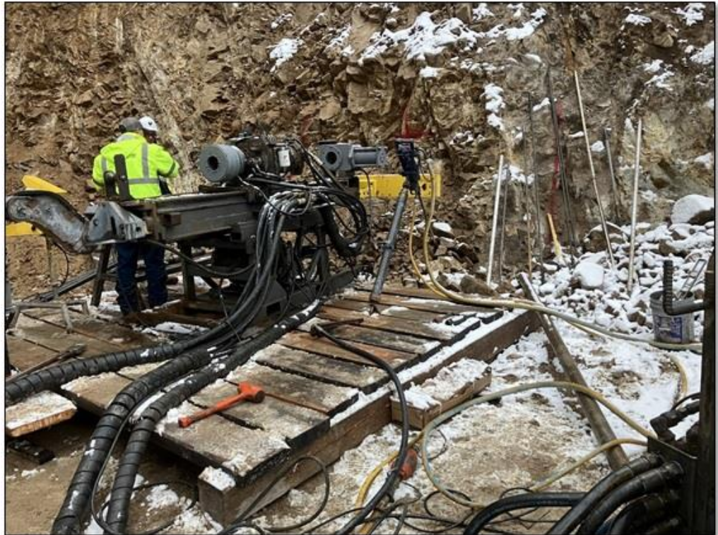
Figure 1: Contract Miner at Face at Washington Mine
