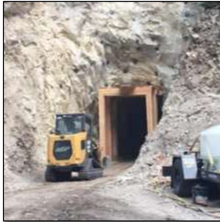
Figure 19: Washington Mine, Idaho – Revitalized Portal
